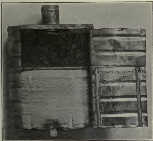
Fig. 104.—Crepe Paper Doughnut Filter Canister.
